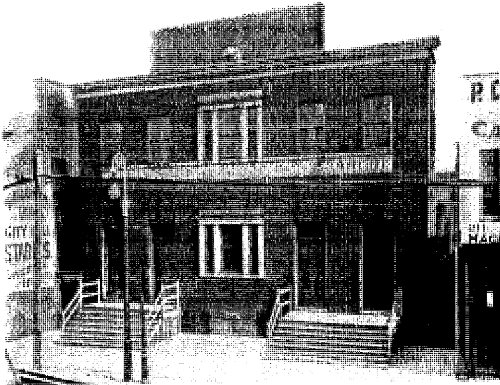
This is the way the old Oliver Hibernian Free School building looked shortly before it was torn down in 1904.
